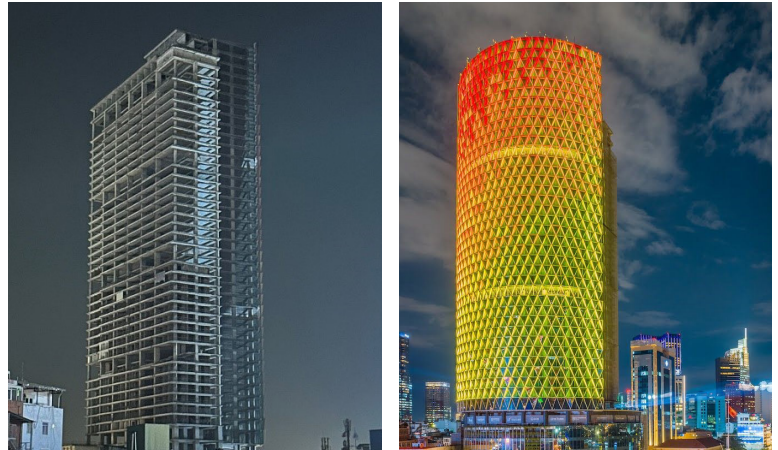
2 sides of the same building – incomplete construction back vs completed and flashy front
